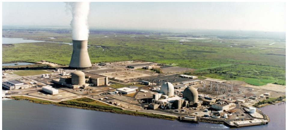
The Hope Creek and Salem nuclear units on Artificial Island in southern New Jersey | BHI Energy
